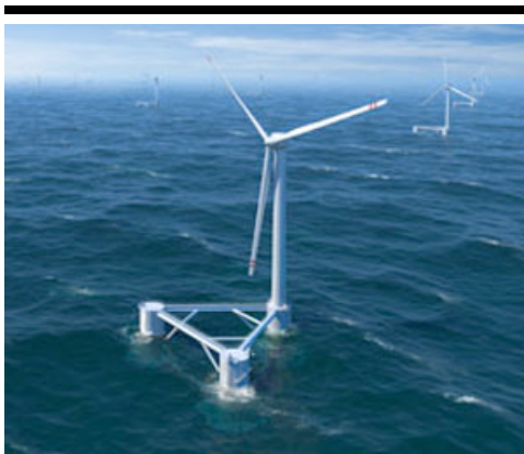
Principle Power is working to develop a 150-megawatt offshore wind power plant using a foundation developed by Marine Innovation & Technology in Oregon.
